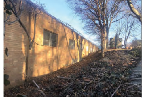
View toward the Cottage along the east wall of the Royal Electric building
